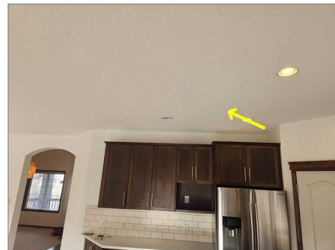
Ceiling staining- No abnormalities detected
